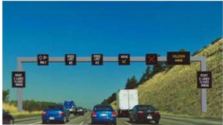
Figure 3 — Variable Speed Limits/Speed Harmonization with Integrated Dynamic Lane Assignment, Seattle, Washington
